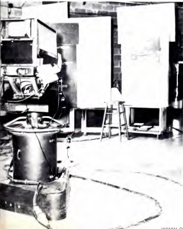
Control panel and console for two-camera remote control system at WHEN-TV, Syracuse, New York. The console is portable and movable between two Control Rooms. Each camera features six "shots" complete with manual hand controls.
